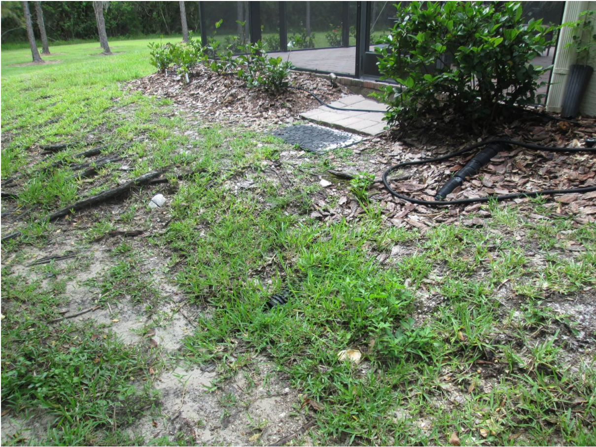
Tree roots and drainage pipe from lanai extending part way down slope
