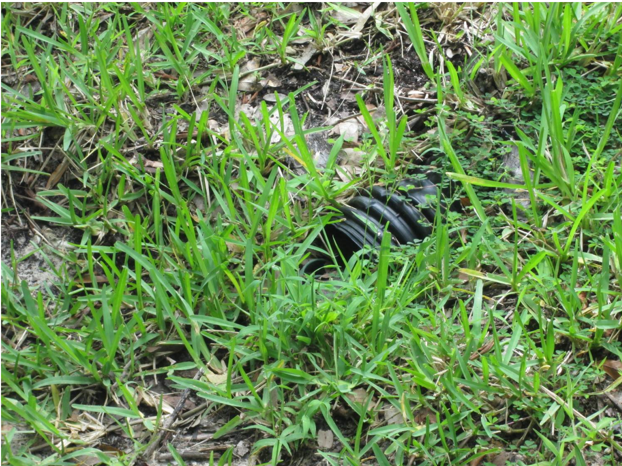
End of drainage pipe from lanai extending part way down slope
